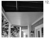
With the carriers installed you can run the panels.
