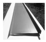
Bend the low end of the panel down into the gutter.
