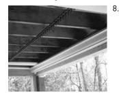
Install gutter to panel height.
