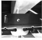
Permanently fasten carriers with screws making sure panel is straight without belly or crown.
