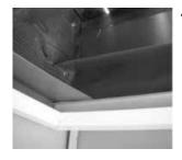
Install Side Cap with a temporary fastener at the gutter end. (remove protective film from Side Cap before installing)
