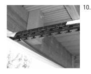
Install remaining carriers with necessary insulators.
