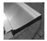
Bend the high side of the panel up to prevent back flow into the G-Channel.
